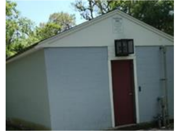
Simmons Pond Pump Station
