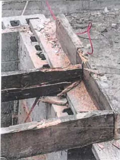
5. Poor framing and damaged joist
