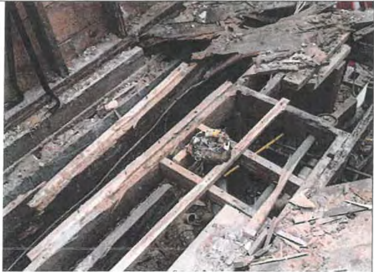
4. Damage & inconsistent framing
