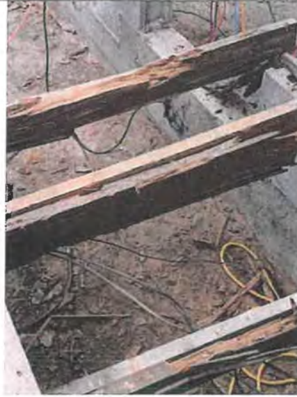
4. Damage & inconsistent framing
