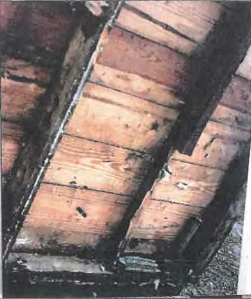
3. Dry rot of floor joist
